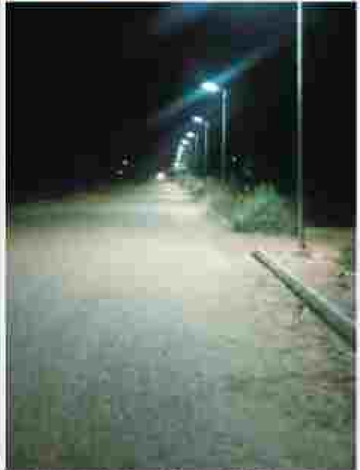
Street lights from Senior Staff Quarters leading to College of Health Sciences
